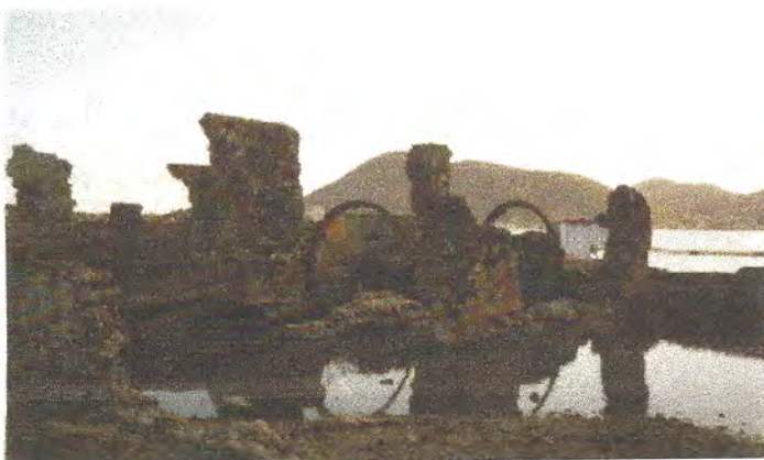
4. After restoration, the ruins of the salt factory could form an educational, historic site for both tourists and islanders.
